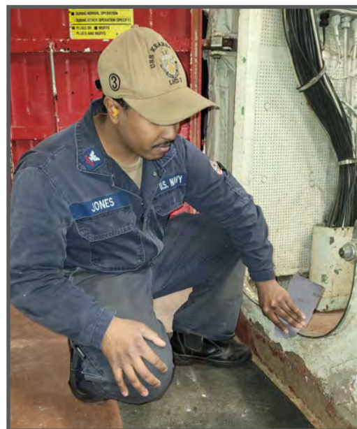
MM2 Jones using a 320-grit abrasive cloth on watertight door knife edge to remove paint rust and corrosion.
