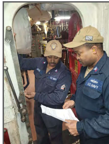
MM1 (SW) Cleon John and MM2 Demetrious Jones conduct preventive maintenance on a watertight door.
