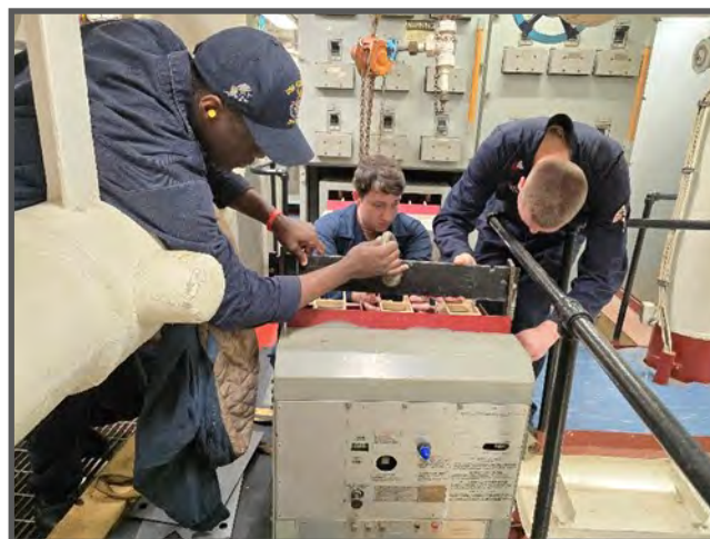
EMFN Michael Adomako, EM3 Williams Hughes and EM1 (SW) Riley Sutliff prepare rigging equipment on number 1S-2S bus tie circuit breaker in preparation for installation in number 1 switchboard.
