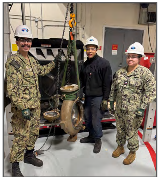
(L-R) BM2(SW/AW) John Pedraza, BM2(SW) Asahiah Grimes, and BM2(SW) Kateri Vizcarra work with the MARMC pump shop to complete jobs. (Photo by Felicia Reid.)
